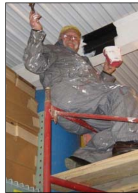
Jon Stahley painting in Station 7
